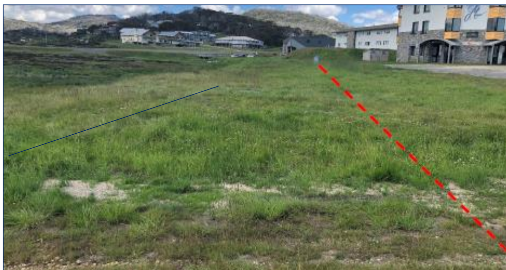
Figure 3 | Alignment of drainage line (red dash) and conveyor between Village 8 Chairlift and Perisher Creek (Source: Applicant's documentation)
